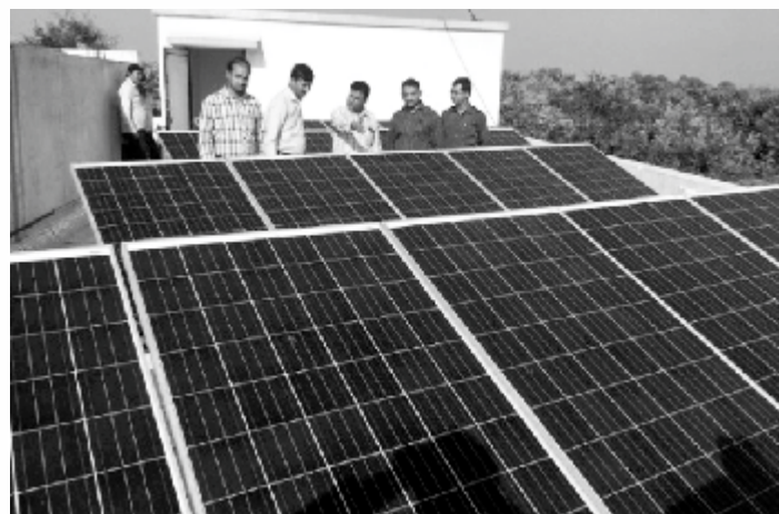
Solar panel at CNG station
